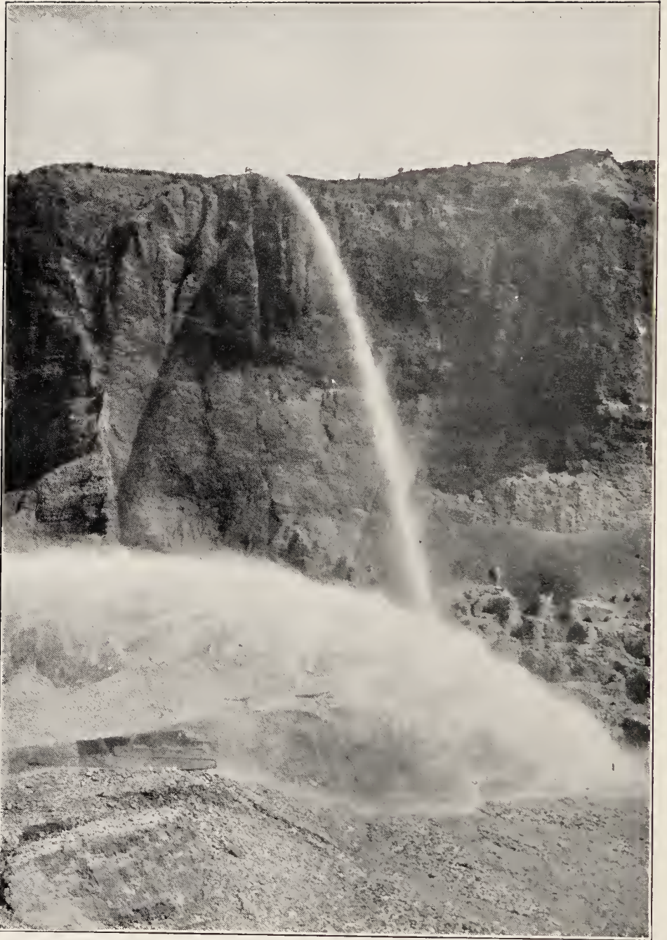
To get the water for washing down the gold-bearing gravel of the Klondike hills, millions of dollars were spent in building ditches, flumes, and pipes from the Tombstone Mountains, seventy miles away.
